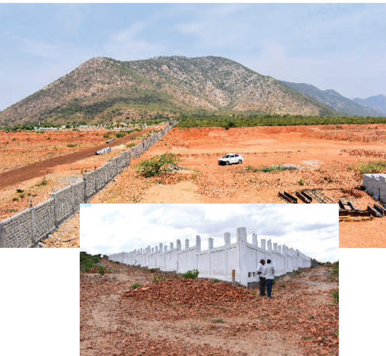
A view of the compound wall of permanent campus
